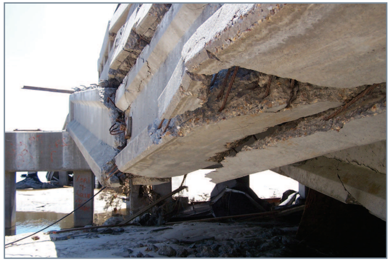
Bridge damage from Hurricane Katrina, September 2005
